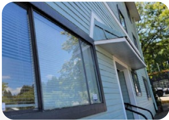
BC Housing's Rialto building
